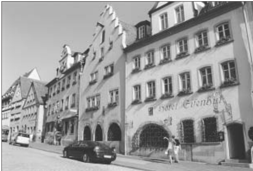
The three buildings comprising the main section of the Hotel Eisenhut (Wallace)
